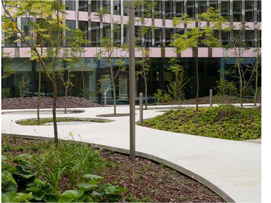
Long span bespoke concrete paving with light colour pigments
